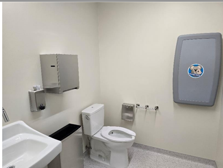
Washrooms are completed and washroom accessories are installed.
