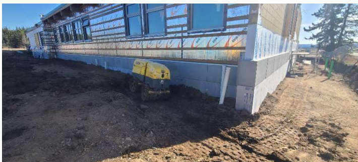
While the finishing progresses on the inside, excavation, drain tile installation, backfill and compaction work progresses outside.
