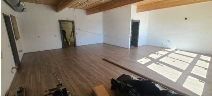
Flooring and a glimpse of things coming together in the 3-5 year daycare room
