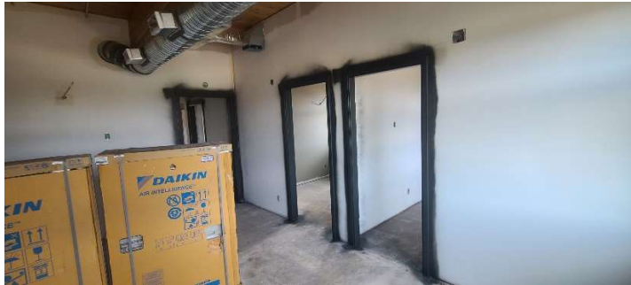
Door Frames are installed and being painted
