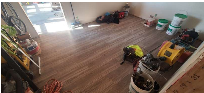
The flooring installed in the shared kitchenette between 0-3 and 3-5 years daycare rooms
