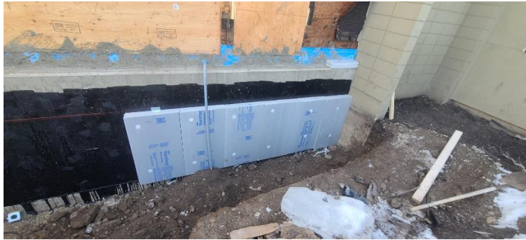
Insulation is being installed on the S side foundation wall
