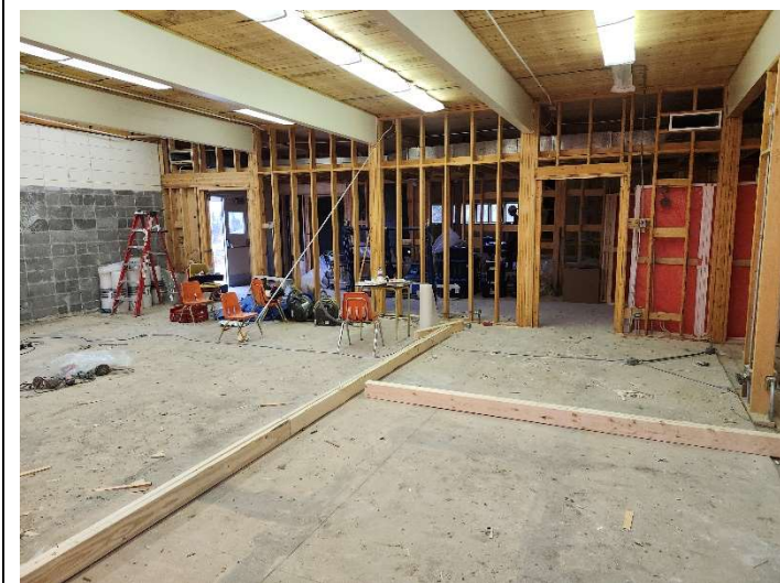
Demolition progress of the S rooms
