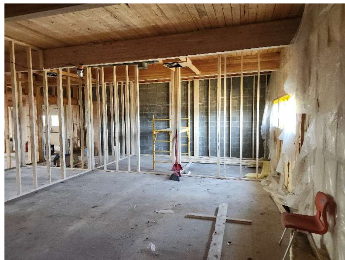
Framing for new offices on the NW Side, previously part of the Home Economics Classroom
