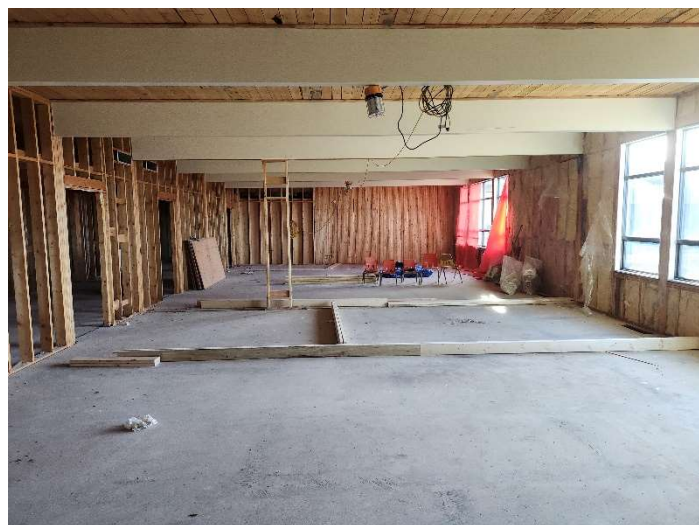
S classroom demolition complete ready for framing.
