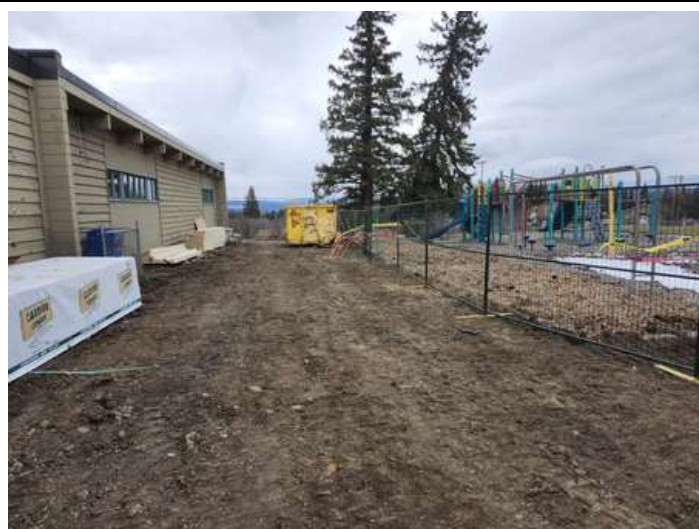
Playground Reinstated and fencing reinstalled along perimeter.
