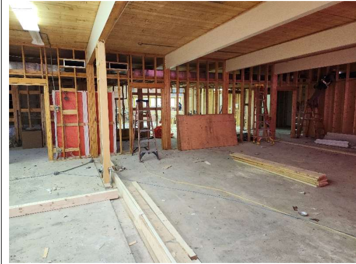
Demolition nearing completion. Some framing material is being staged for the new walls
