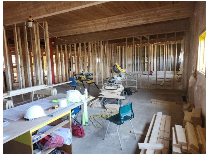
Framing of a new Classroom, looking towards Keefe's Landing Rd.
