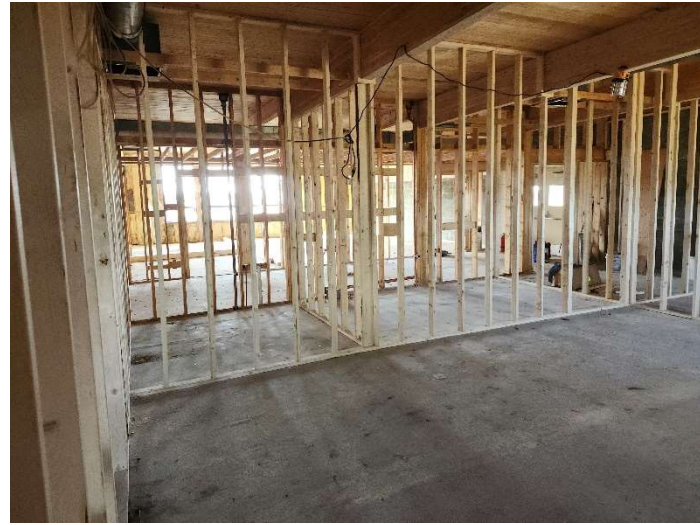
Framing has begun on N side room. Previously this was a computer room, now it is framed for 2 new washrooms
