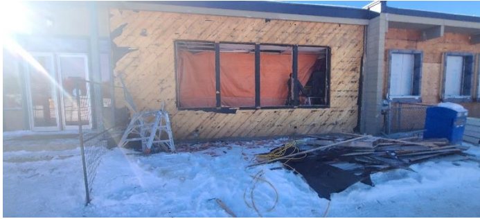
Windows were removed in preparation for new fiberglass window installation
