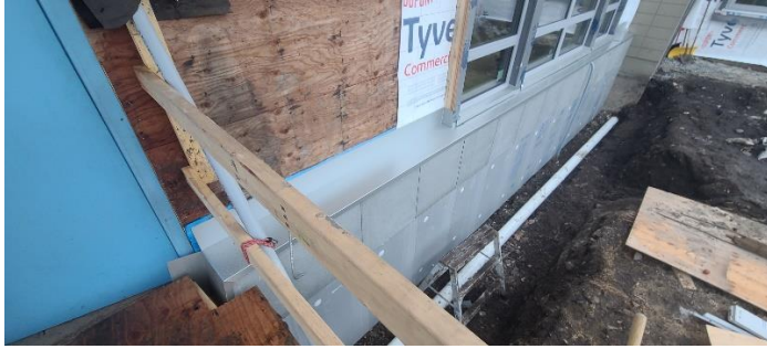
Foundation insulation and new drain tile was installed along the S side of the building
