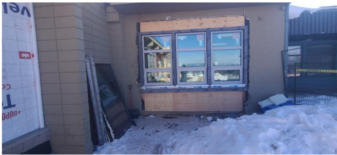
Classroom windows that were replaced
