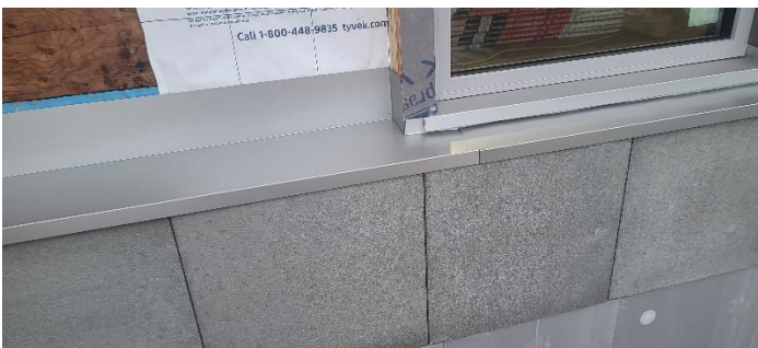
Concrete faced insulation (CFI) was installed for the top 2 feet. It provides a finished surface above ground level.
