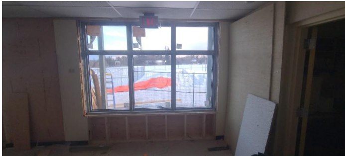
Library Exit door was replaced with a bank of windows
