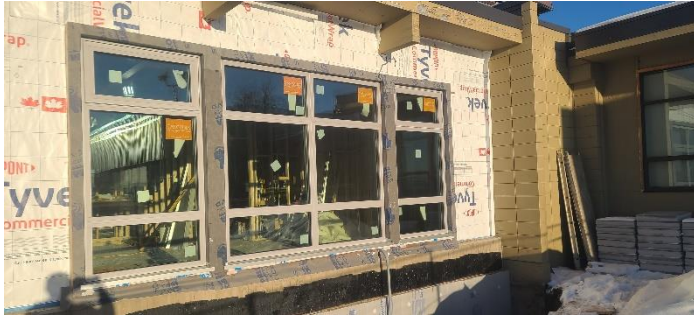
New Windows were installed throughout the daycare, library and one classroom.
