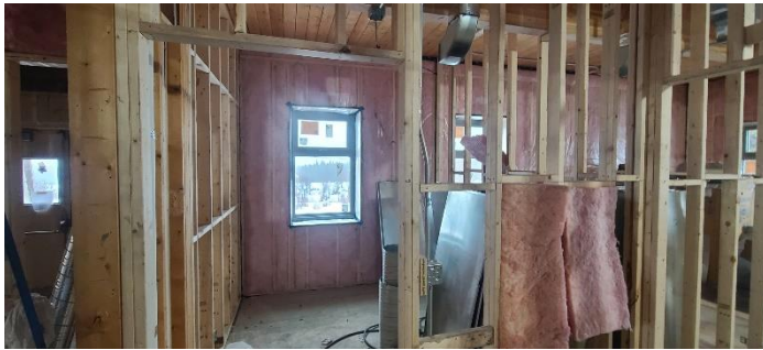
New windows in the cinder block wall will bring natural light in to new offices
