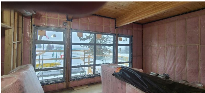
New insulation and windows installed
