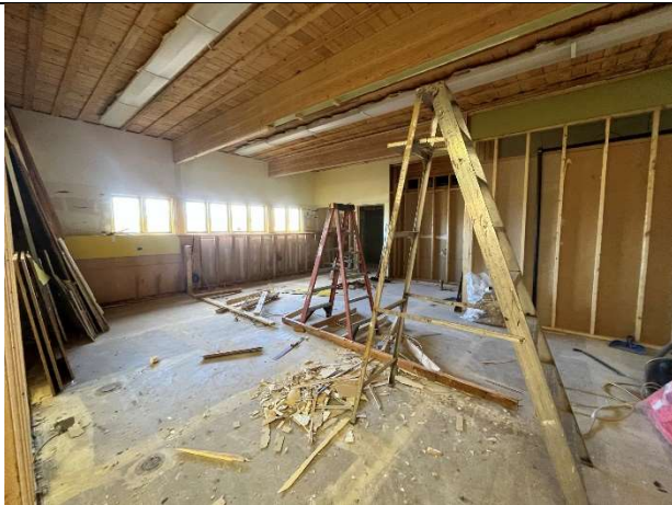
Following the completion of hazardous materials abatement, demolition of the Computer Room has begun
